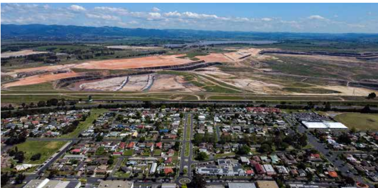
View over the town of Morwell towards the Hazelwood mine site. Image supplied by Friends of Latrobe Water.
